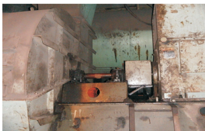
Fig 1: Combustion Air Fan in Wire Rod Mill Department (VSP).
