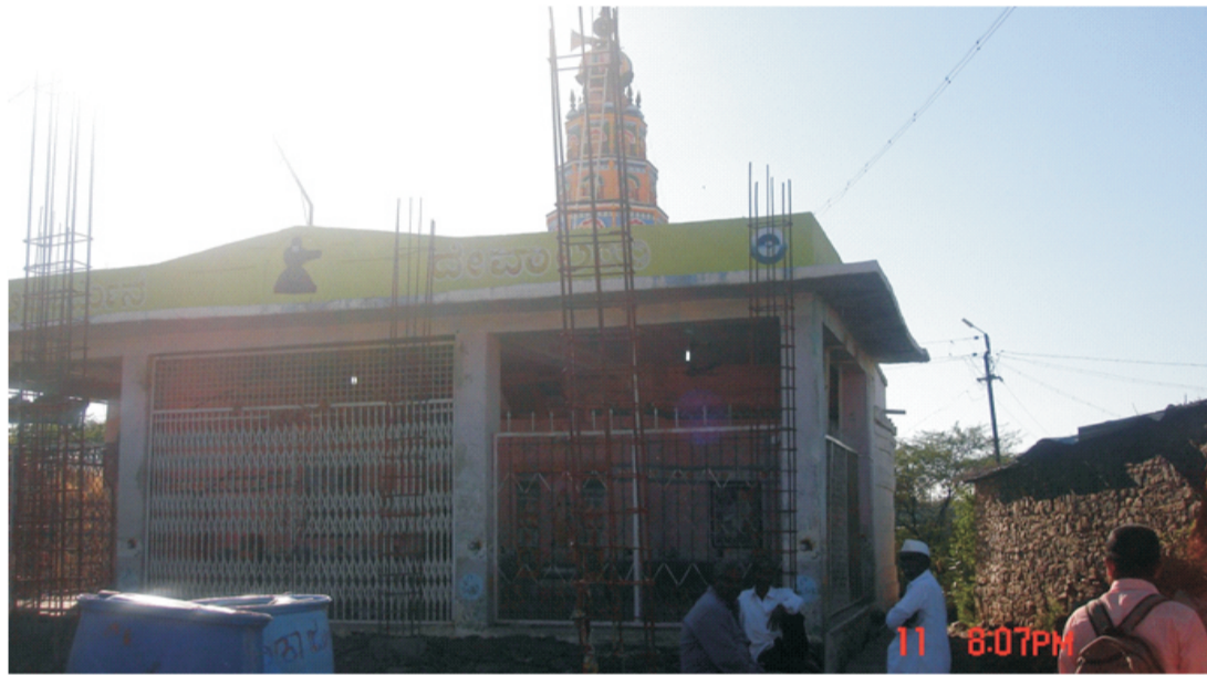
Mallikarjuna Temple at Bhodan
