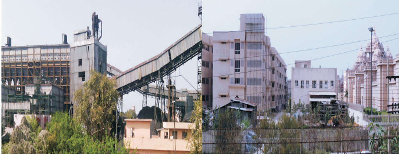
Rajghat Thermal Power Plant
