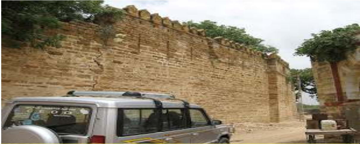
Inner fort wall
