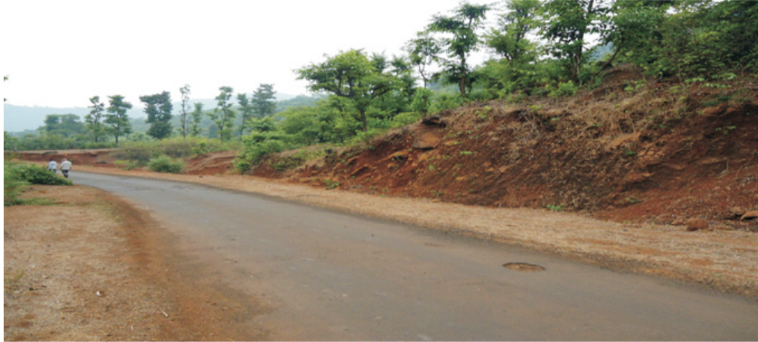
Plate 3 : Construction of Road (Location – Marleshwar)
