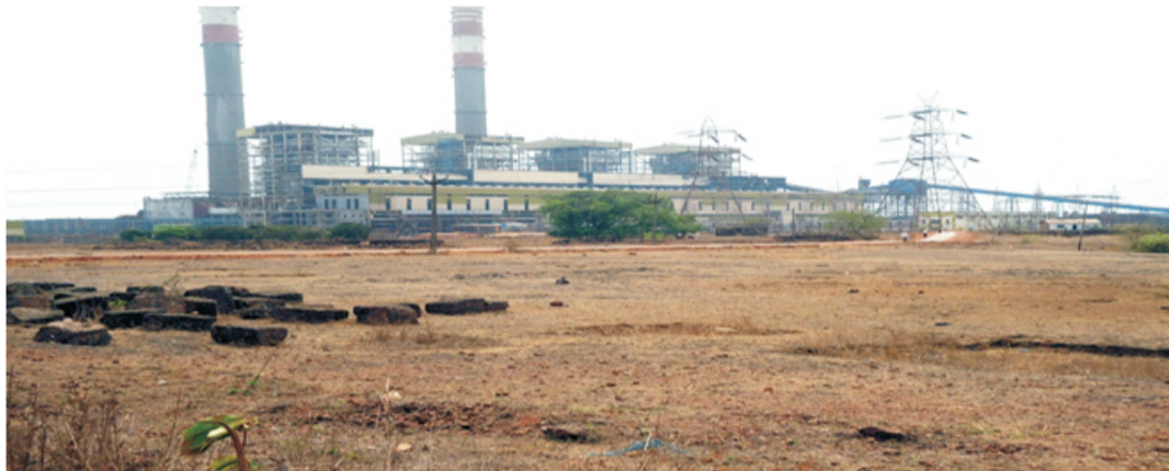
Plate 7: Thermal Power Plant Over Lateritic Terrain (Location – Jaigarh)
