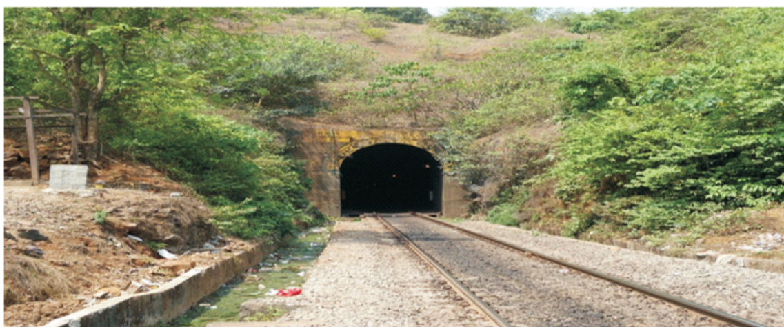
Plate 5: Construction of Railway Tunnel (Location – Karbude)
