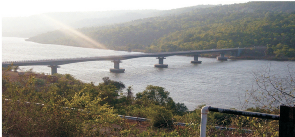
Plate 4: Construction of Bridge Across Shastri River (Location - Bhatgaon)
