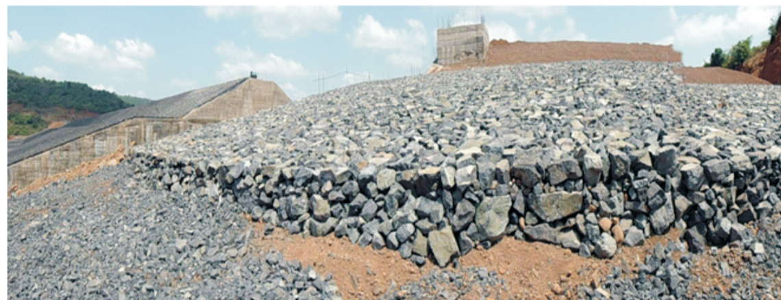
Plate 2: Pitching of a Dam (Location- Kuchambe)
