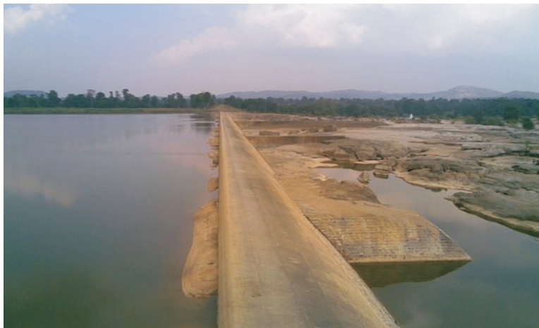
Fig. 1. A View of Bheemgarh Dam
